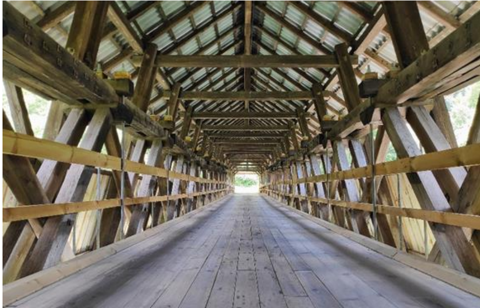
Figure 1. – The Gau system bridge over the Sava River where such material was used.
