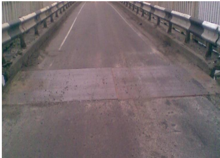
Fig. 1 – The deformation seam of gravitational type is arranged
